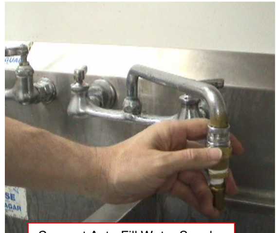
Connect Auto-Fill Water Supply Hose to machine and faucet
