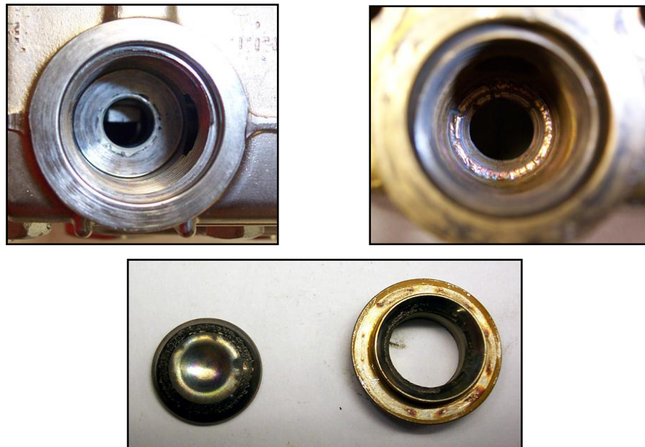
Figure 5-2. Inspect Manifold and Old Valves
