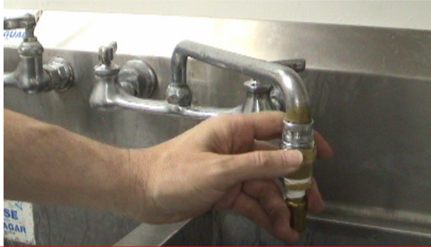
Connect the Auto-Fill Water Supply Hose to a faucet and turn on the water
